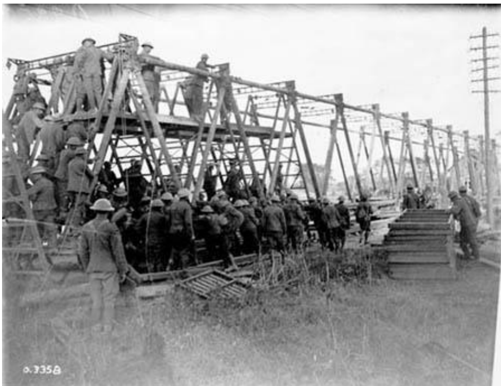
Canadian Engineers preparing bridging for the Canal du Nord Crossing
